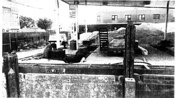
PROJECT: East West Properties, LLC-Ashland Ave PHOTOGRAPH #21 DATE: 9/26/23 VIEW: South DESCRIPTION: Backfilling Tank Excavation with Gravel
